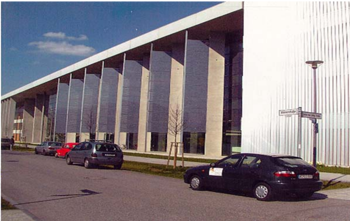
PV-Facade of the Center for Bio- and Environmental Technology, 14 kW p , 1998, AstroPower Apex-cells, Modules made by SOLON
