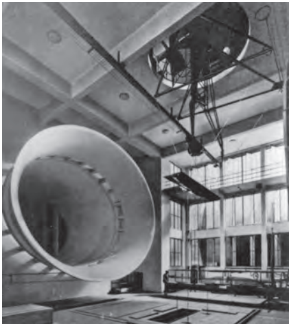
View of the measurement hall of the Great Wind Canal and the discharge nozzle and the six-component scale on the top floor
